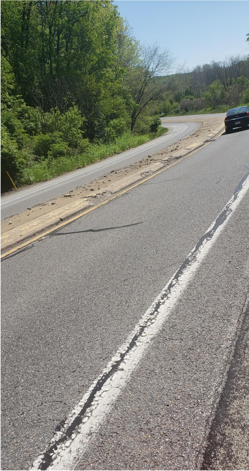
PICTURE #2: MONTOUR RUN ROAD WESTBOUND AND EASTBOUND LANES
