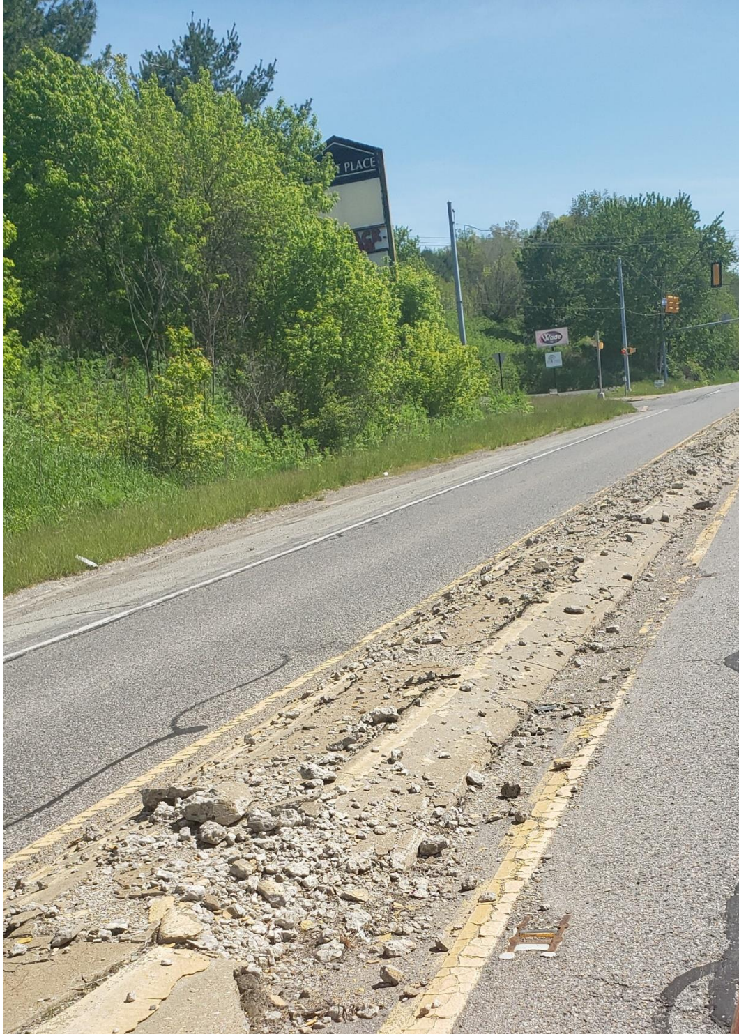
PICTURE #1: MONTOUR RUN ROAD WESTBOUND LANE AND ROADWAY MEDIAN
